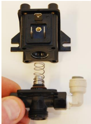
Step 4: When separating spray solenoid, note the piston and spring position in the piston shaft.
